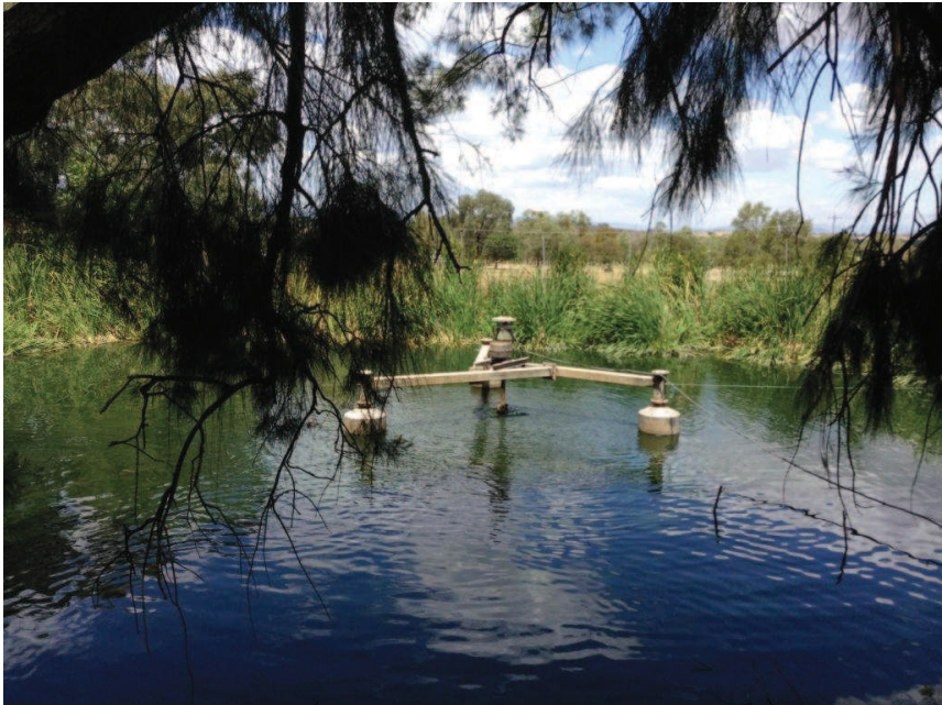
Plate 17: View of Waste Water Aeration Pond within Lot 12 in DP 623431
