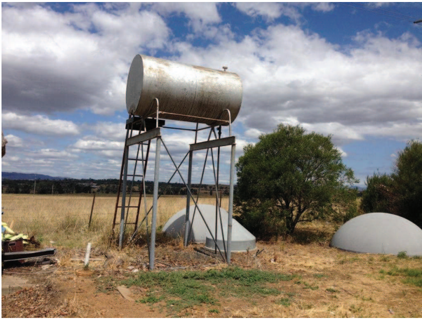
Plate 12: View of Above Ground Storage Tank at the rear of the Prime News Station
